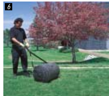
6 Roll sod with heavy roller.
