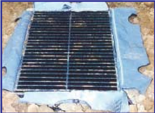
installed Siltsack held in place by grate.
